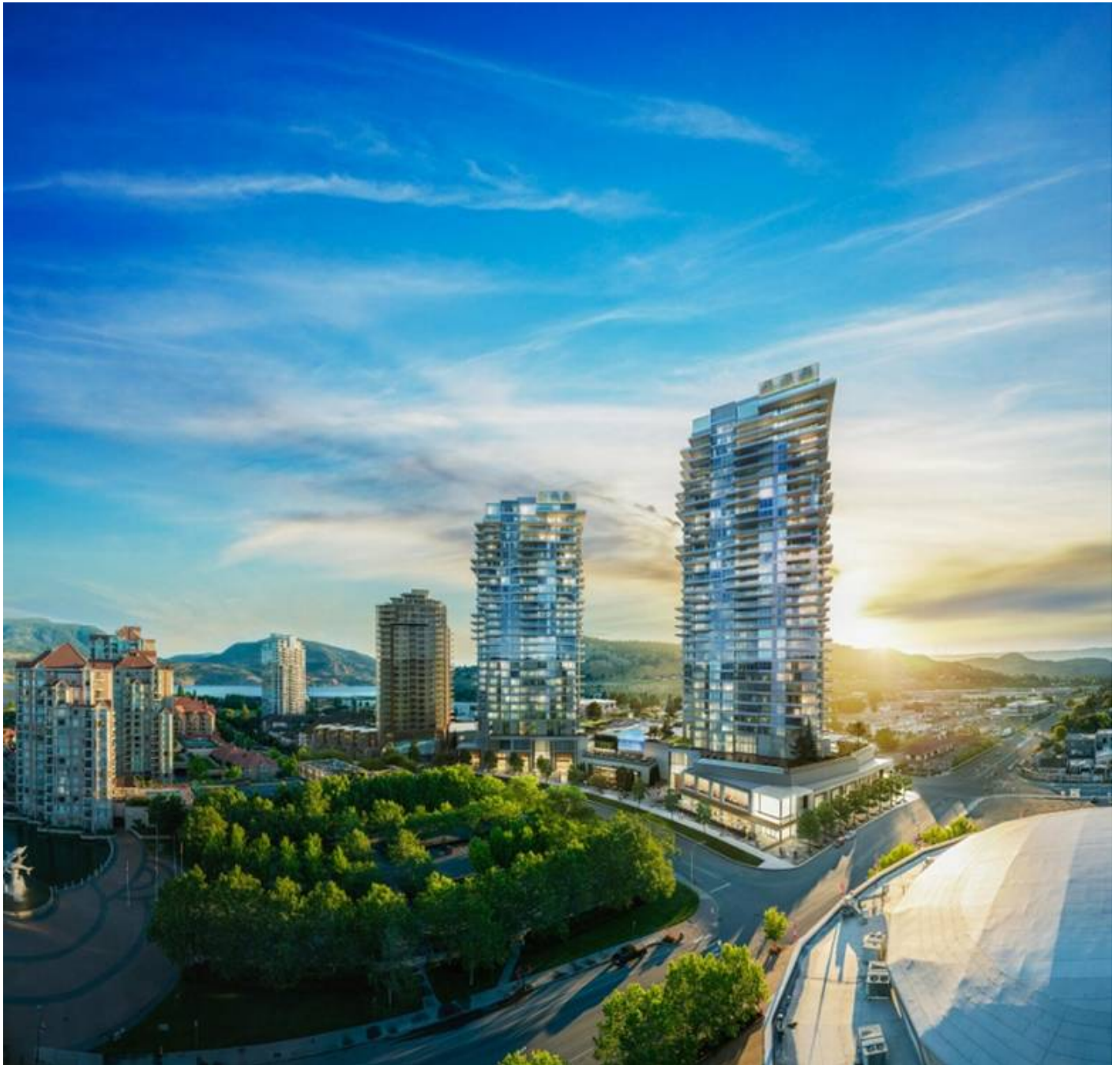
The condo development One Water Street in Kelowna, B.C.
